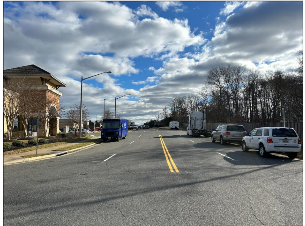
Galveston Court restriping
