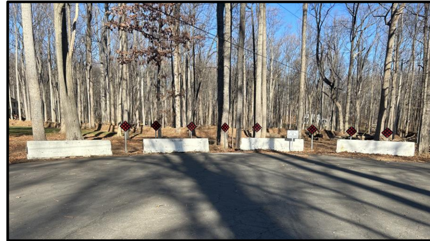
Spring Lake Drive Object Markers and Barricade
