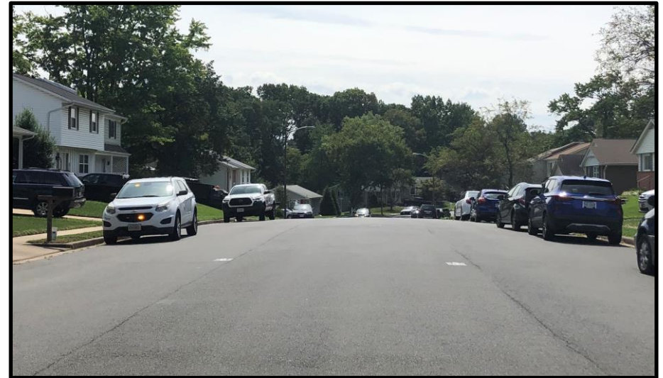
Loop Detectors on Valleywood Drive
