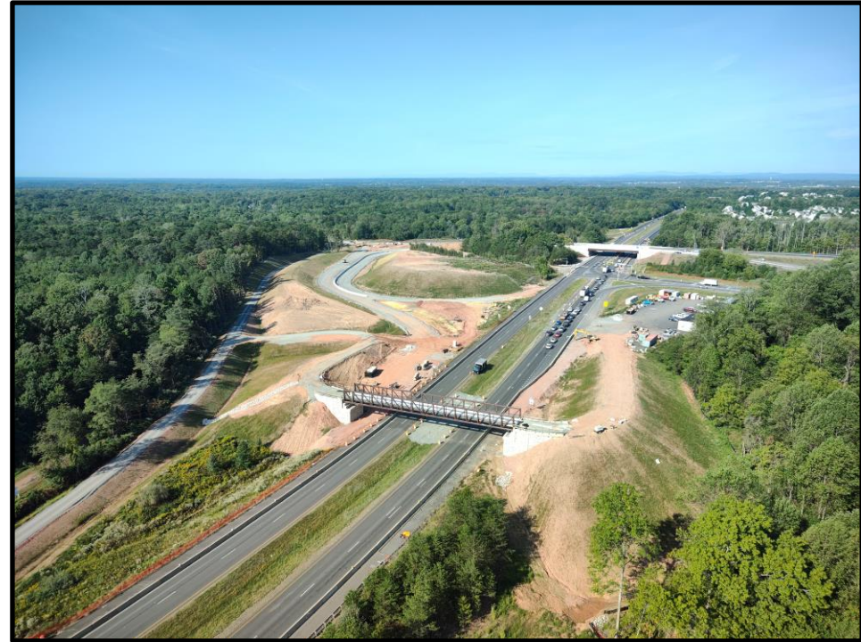
Brentsville Road Pedestrian Bridge
