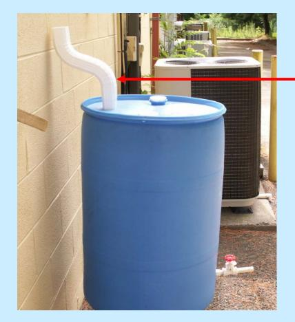
You can connect the downspout directly to the barrel using the 2x3" elbows.
