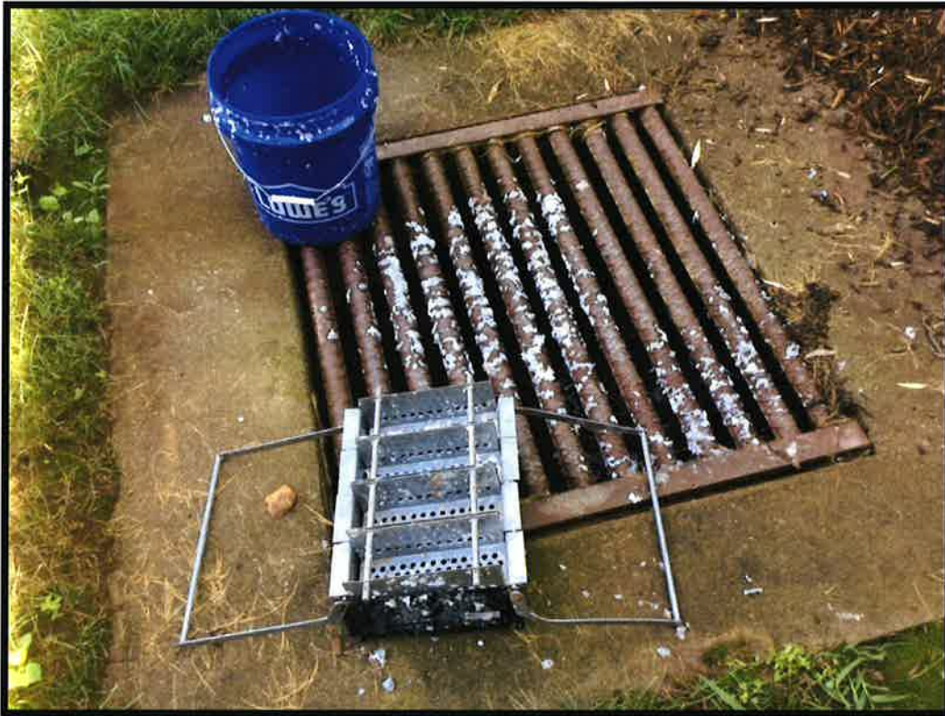
Figure 1: Photo of Discharge.
