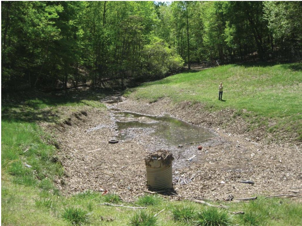
Facility 28. Upstream view of existing sediment basin with riser structure
