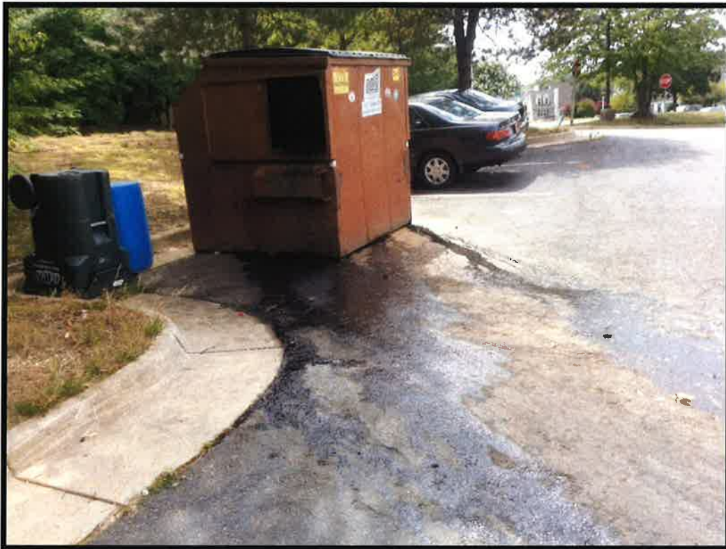
Figure 1: Photo of Discharge.
