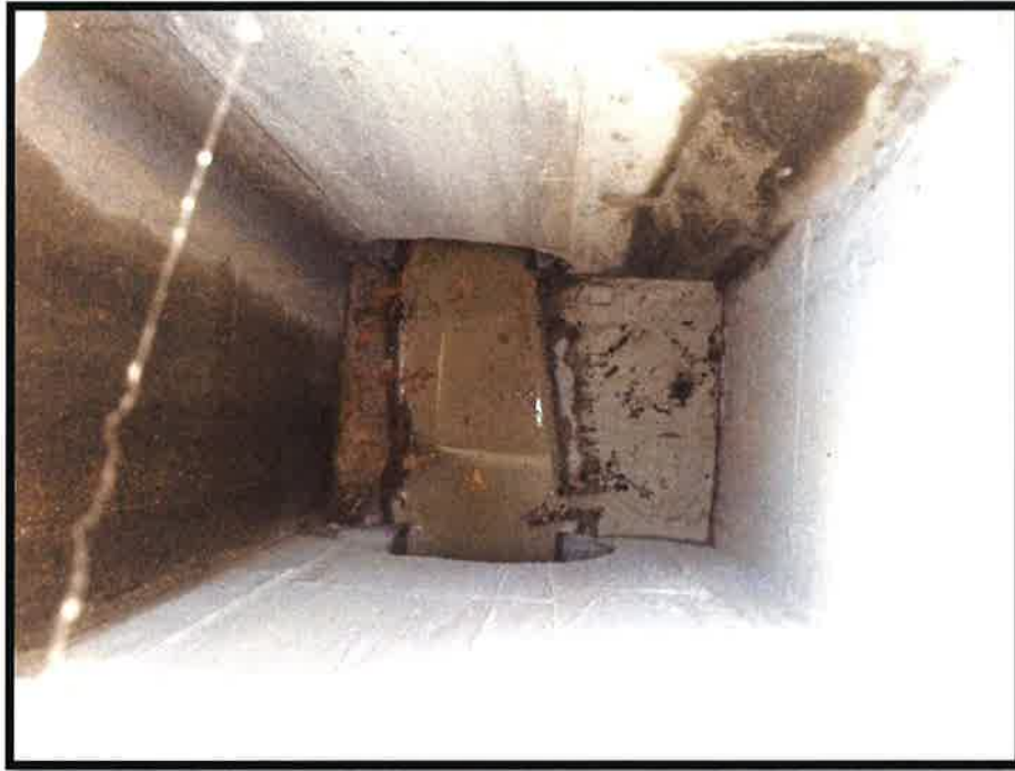
Figure 1: Photo of Discharge.
