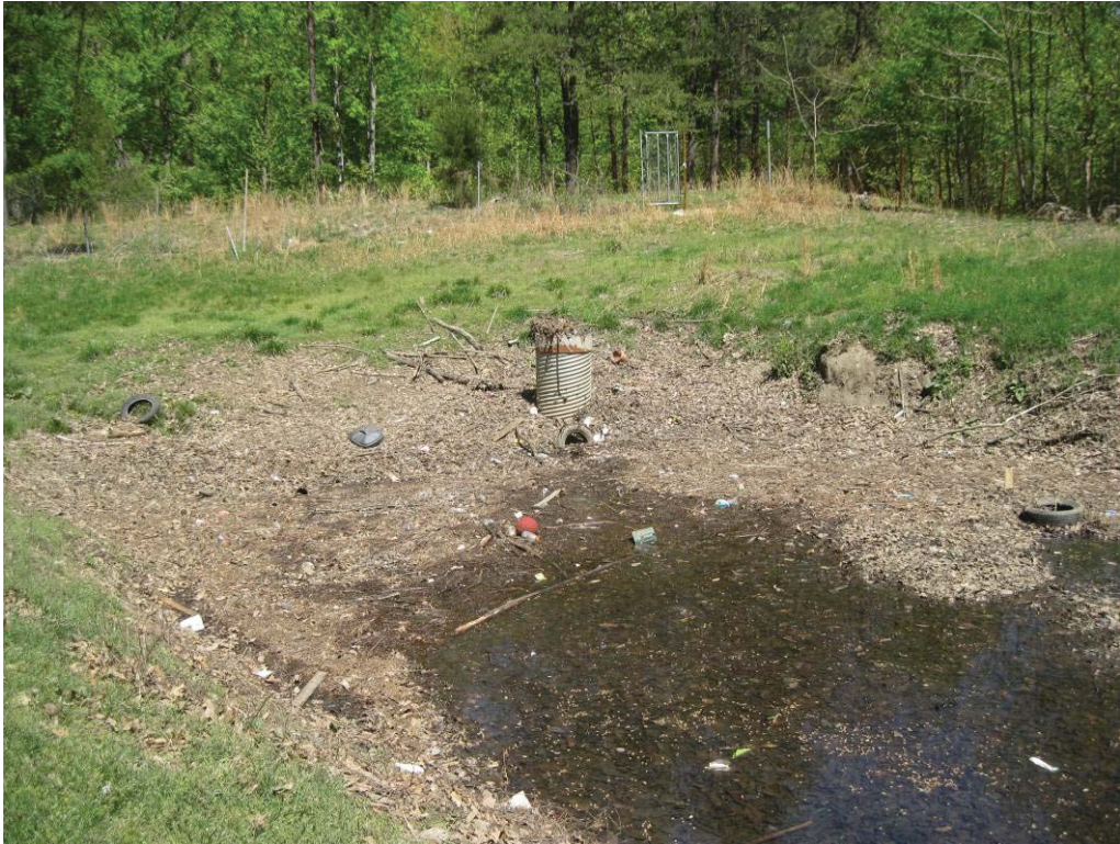
Facility 28. Downstream view of existing sediment basin with riser structure
