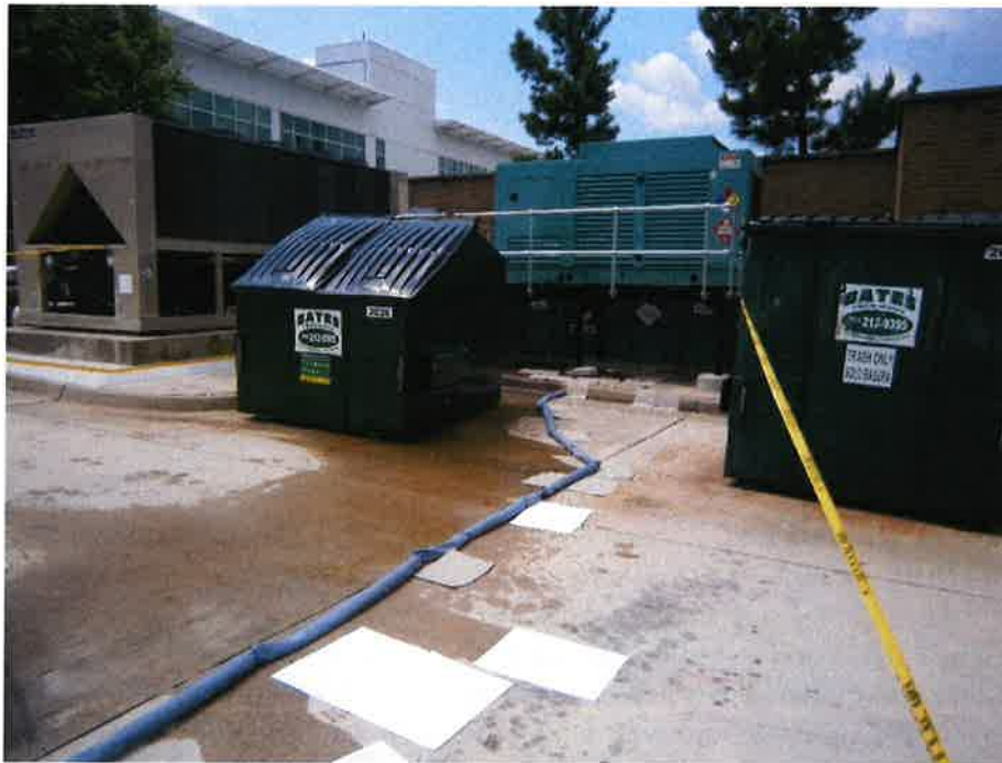
Figure 1: Photo of Discharge.
