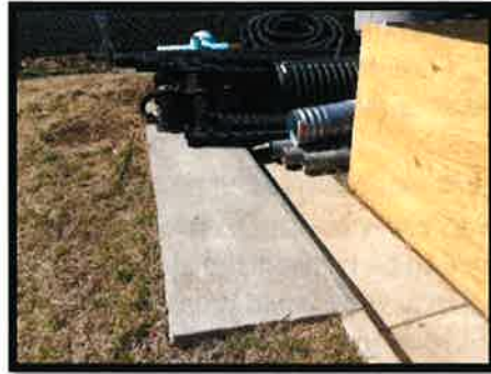
Materials- stacked over structure
