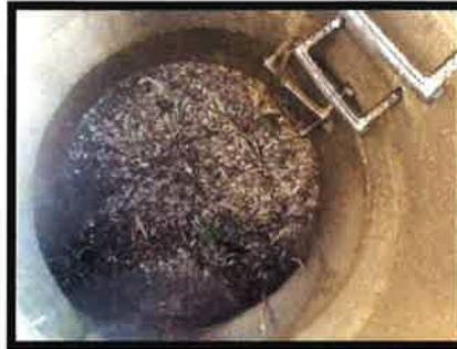
Figure 1: Photo of Discharge.
