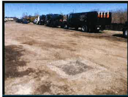
Tar stain under sprayer truck
