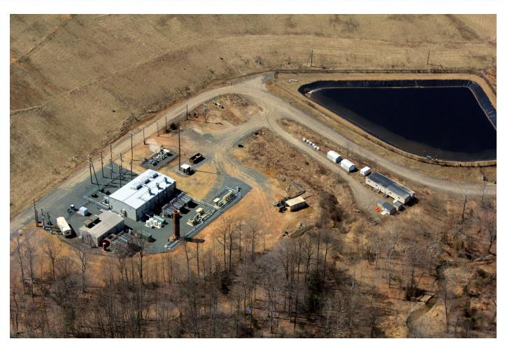
The landfill gas is converted to electricity to produce 6.7 megawatts of power.
