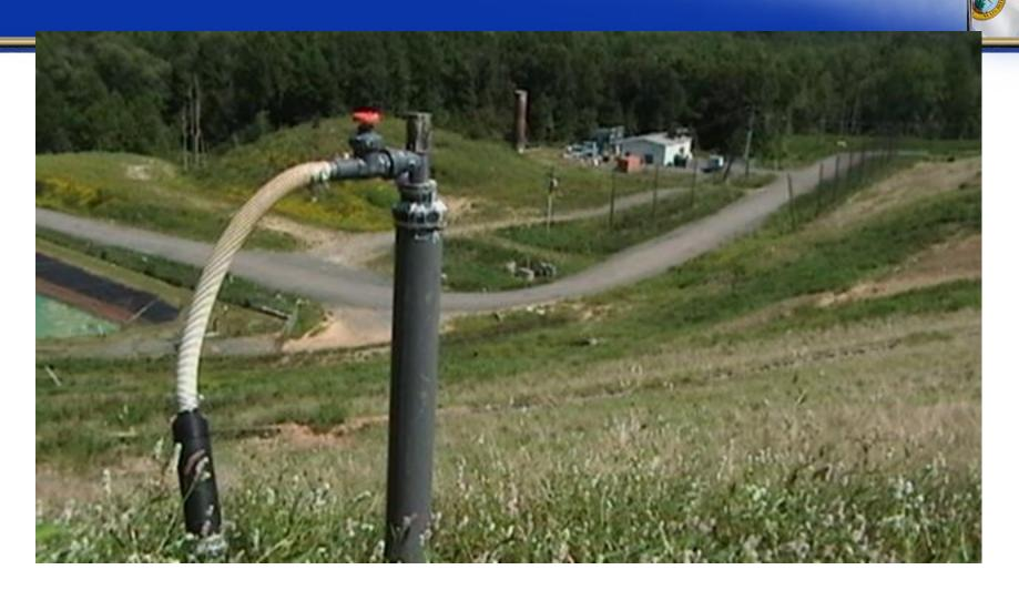
The landfill has over 100 extraction wells for collection of landfill gas.
