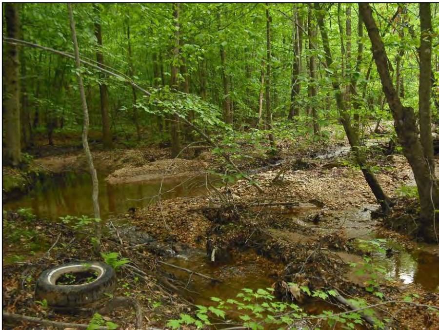
Photo 30: Channel widening along Reach 630-D.
