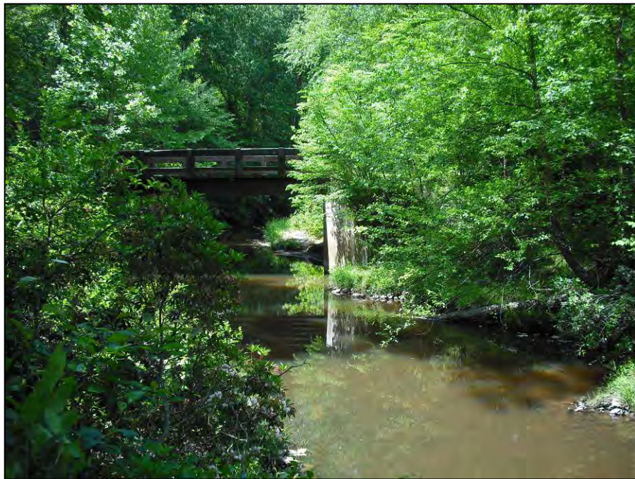
Photo 9: Access road bridge in Prince William Forest Park, Reach 615-C.
