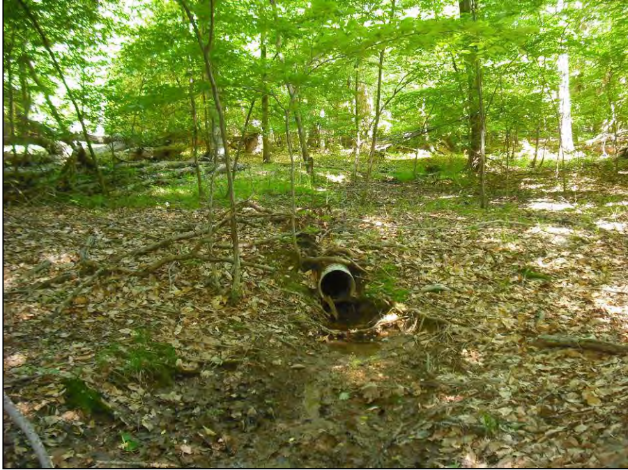
Photo 408: Pipe outfall, downstream of Park Entrance Road, on Reach 645-D.
