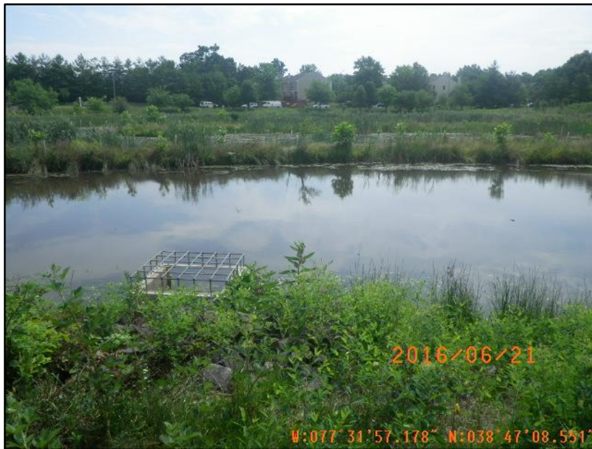
Figure 3–1. Example of stormwater facility conversion. Dry Pond facility (top) converted to constructed wetland with riser structure (bottom). Photo credit Prince William County
