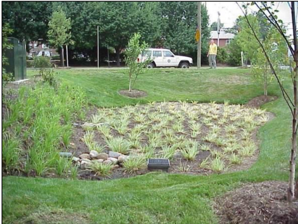
Figure 3–2. Example of bioretention facility. Photo credit Virginia Water Resources Research Center
