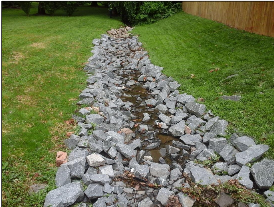
Figure 3-3. Example of outfall rip-rap stabilization. Photo credit Versar.
