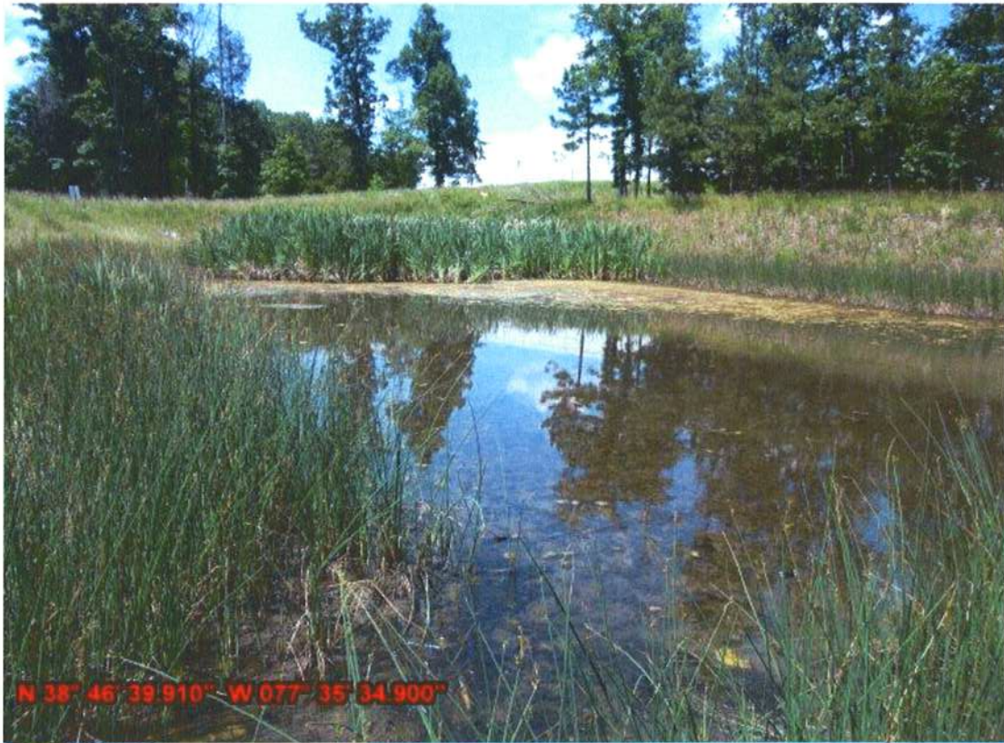
Photo 1: Wetland covers a significant portion of this dry basin with 12” of water over the entire basin
