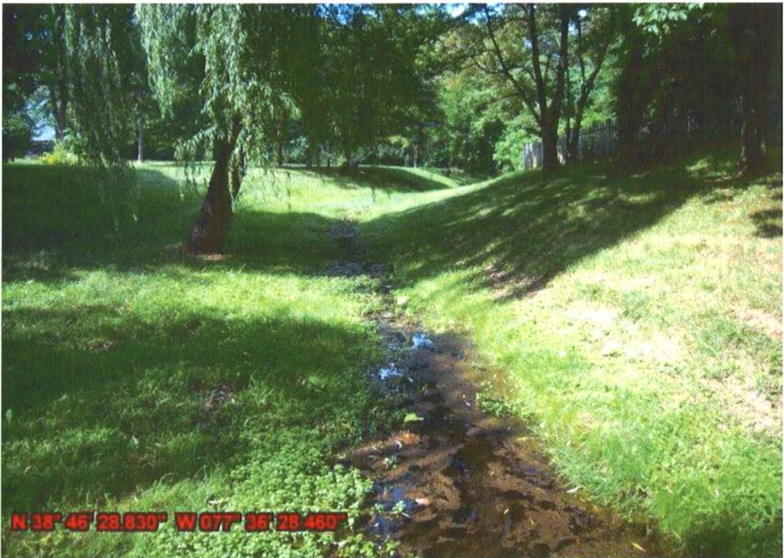
Photo 2: Poorly draining grassed drainage channel is routinely mowed by adjacent landowners, note high algae load in channel
