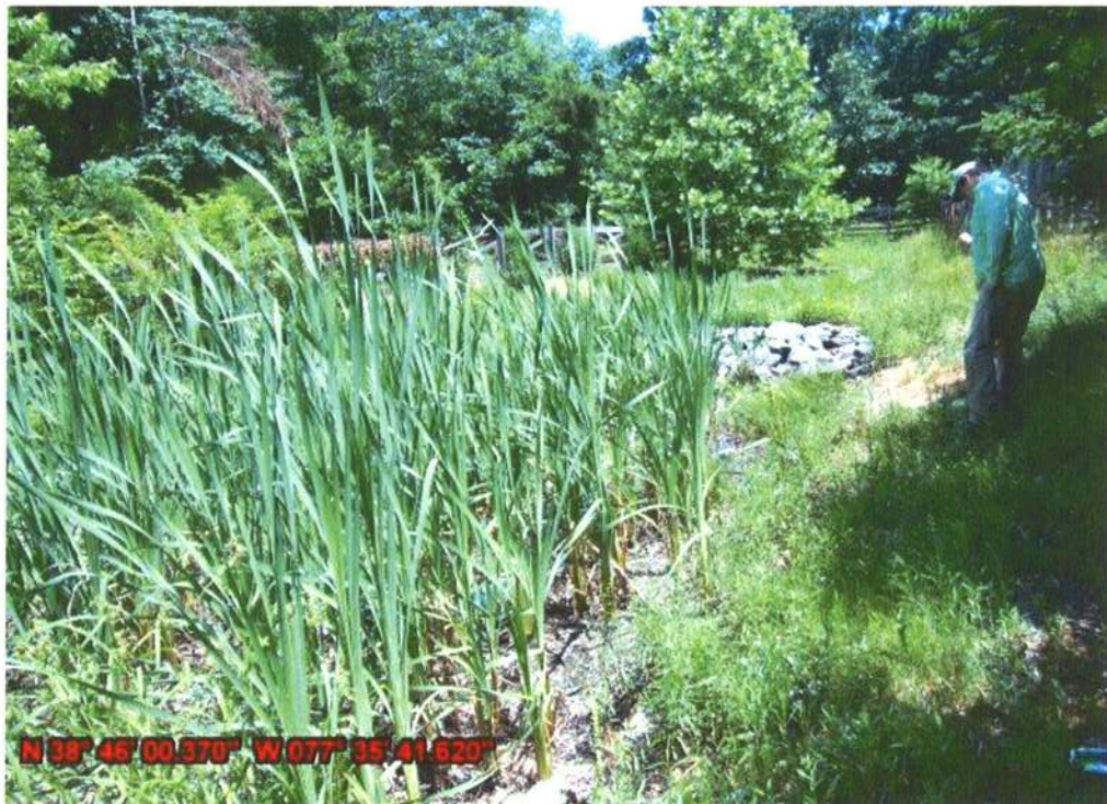
Photo 1: Forebay ponded and supporting wetland vegetation
