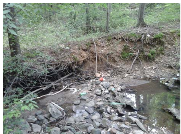
Highly eroded channel with steep banks, surrounded by tree cover.
