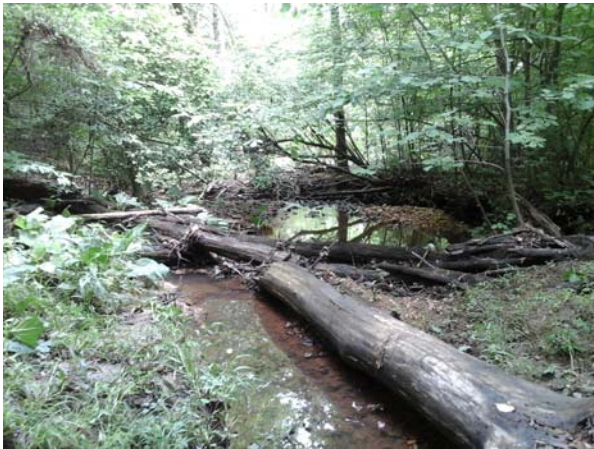
Downstream view of the stream channel, heavily wooded area is visible and minor erosion present.
