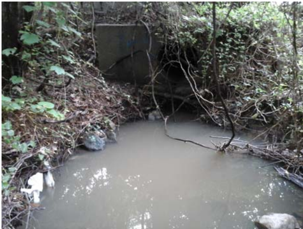
Upstream view of the outfall pipe with plunge pool directly downstream of pipe opening.
