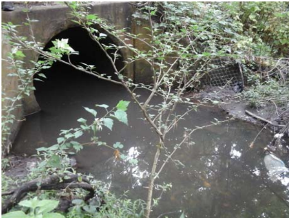
Submerged outfall pipe with flow present surrounded by shrubs and trees.
