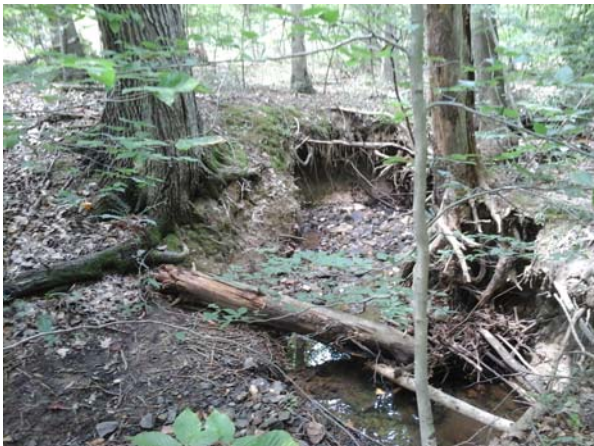
Outfall channel just downstream of the pipe. Severely eroded banks with large trees surrounding the channel.
