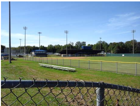
View of existing grassy swale
