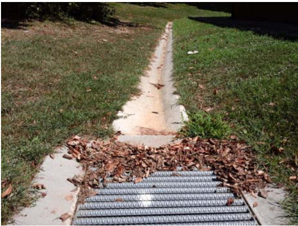
Concrete channel to be improved, west side
