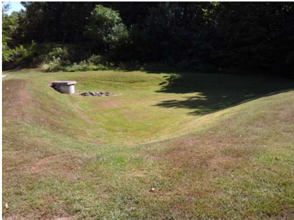
Existing dry detention facility at Logan Park
