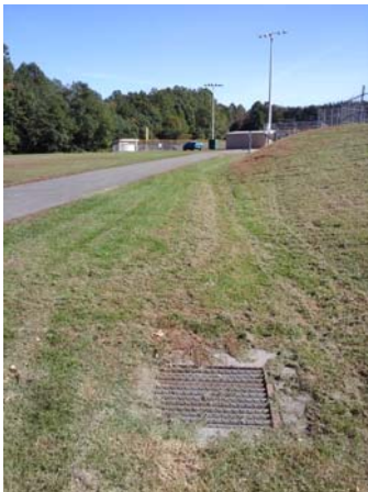
View of drainage to proposed bioswale
