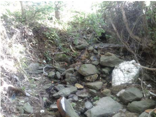
View of outfall and receiving channel
