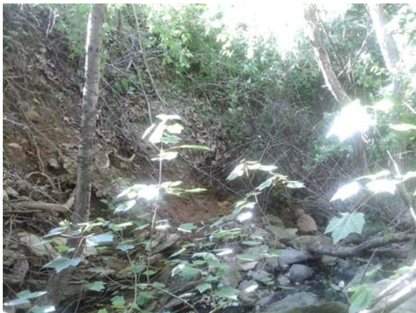
View of outfall and receiving channel
