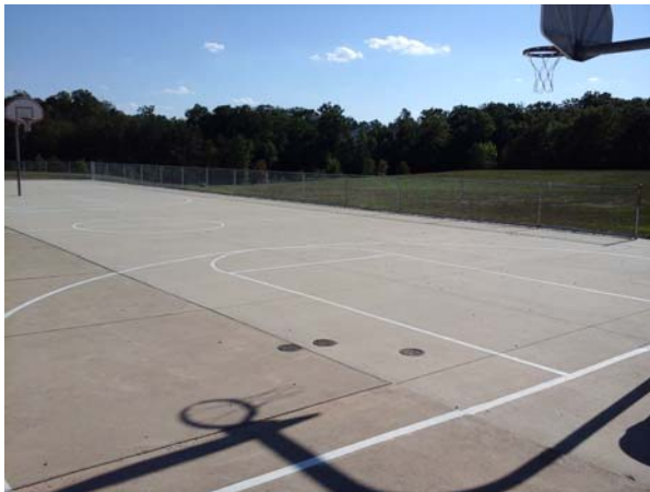
Impervious play area in drainage of potential new BMP
