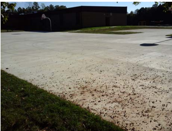
Concrete pad on north side of elementary school
