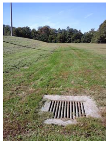
Footprint of potential bioswale leading to yard inlet
