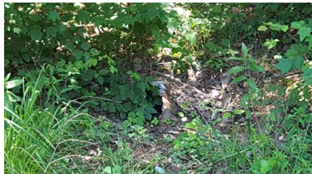
Corrugated pipe in berm of old dry pond facility
