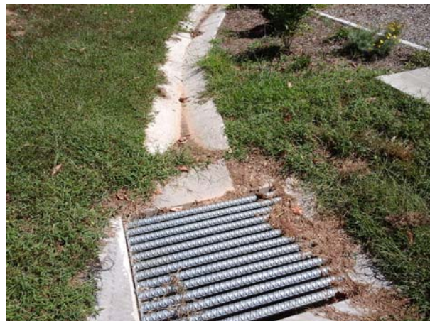
Concrete channel to be improved, east side
