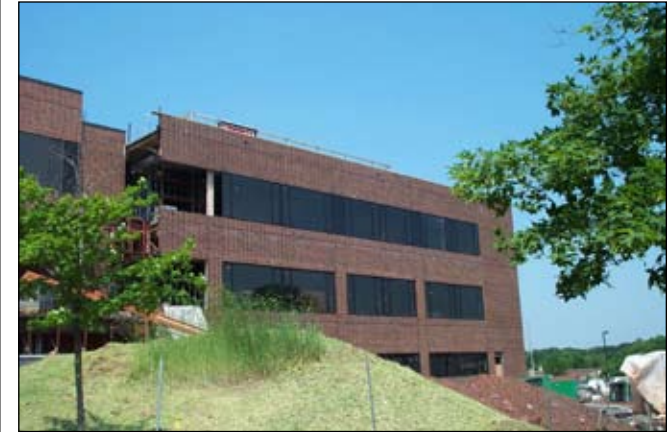
Construction of the Judicial Center Expansion
