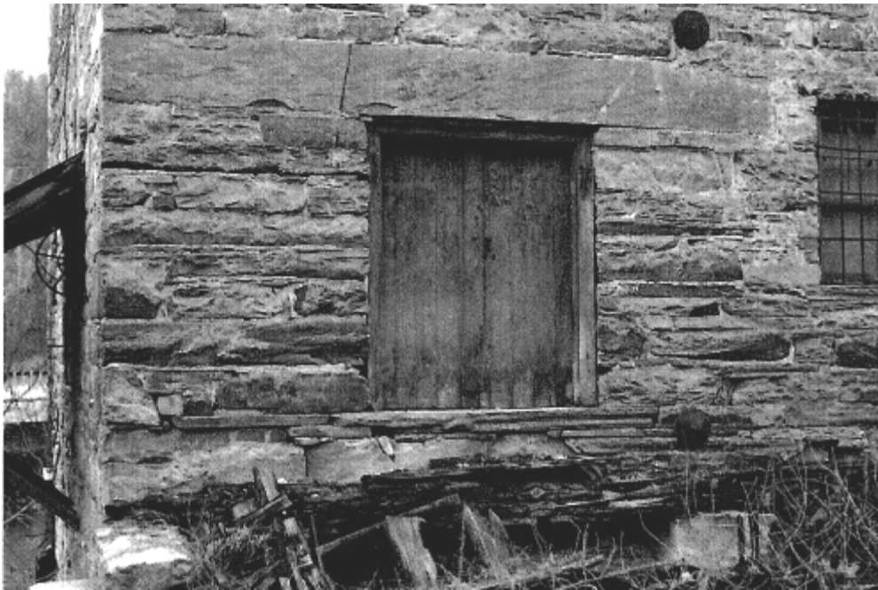
Fig. 14. Entrance, second floor, north side. Photo, Nov. 1980.
