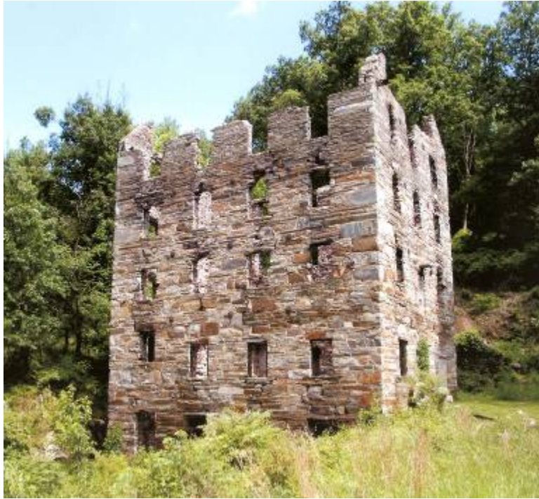
Ruins after the fire
