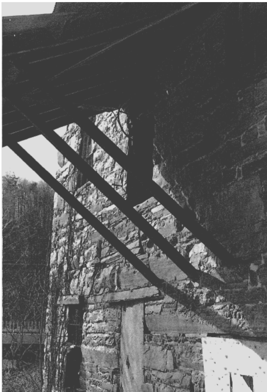
Fig. 13. Canopy with loading entrance, east side. Photo, Nov. 1980.
