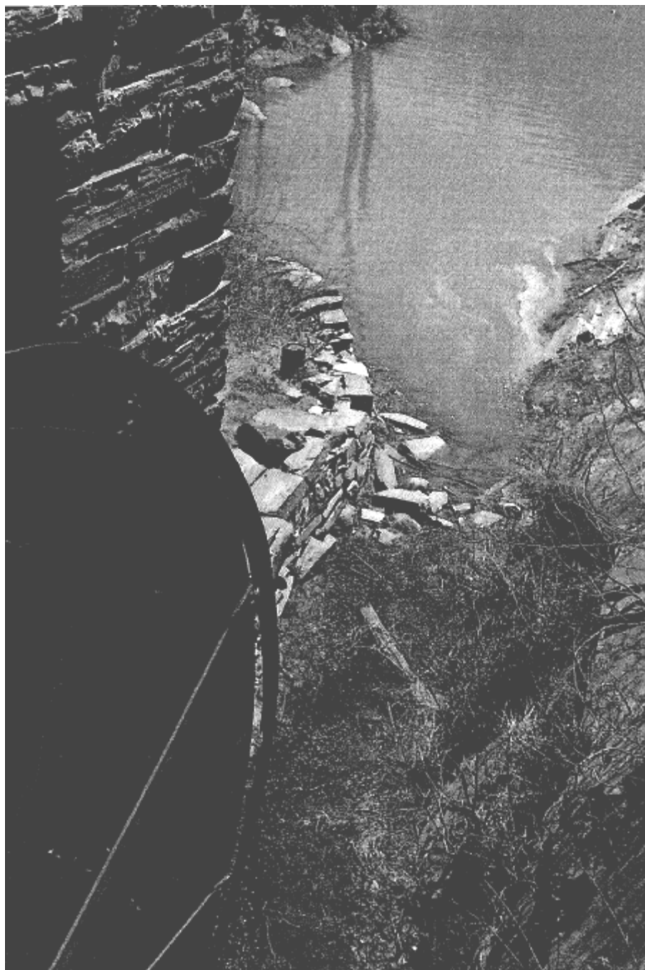
Fig. 16. Tailrace and wheel. Photo, April 1979.
