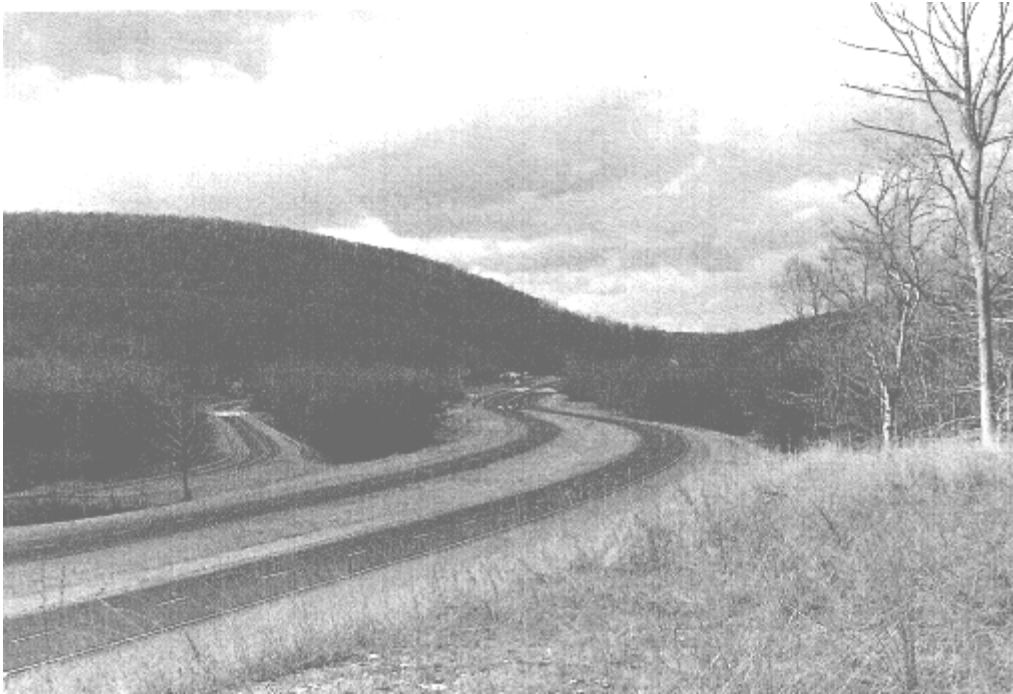
Fig. 6. Thoroughfare Gap. Photo taken from the east. S.R. 55 on left, I-66 on right. Roof of Beverley Mill visible in background, right of I-66. Nov. 1980.
