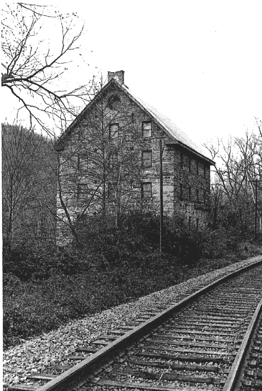
Fig. 12. Mill, east side with railroad in foreground. Photo, Nov. 1980.
