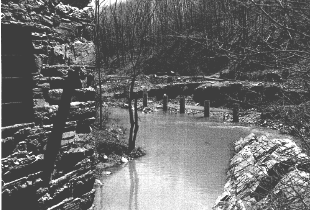
Fig. 17. Broad Run south of the mill, showing bridge pylons for I-66. Photo, April 1979.
