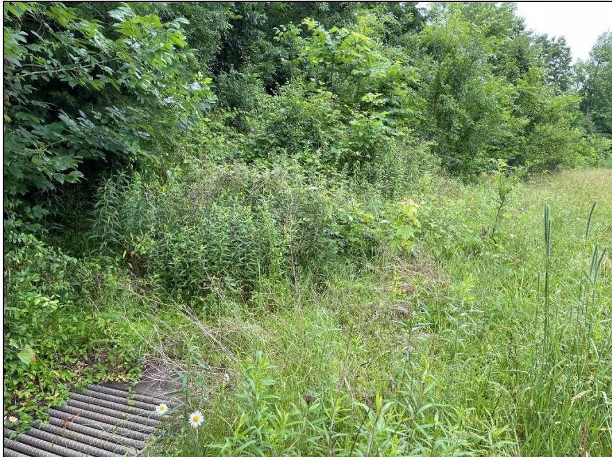
Photo 5: Storm Sewer and Steep Grade Along West Side of Devlin Road, Looking North.
