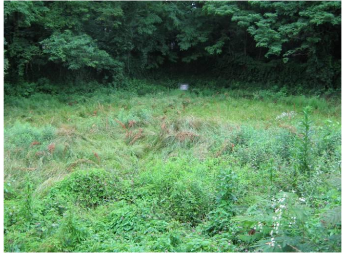
Overview of SWM facility from access gate
