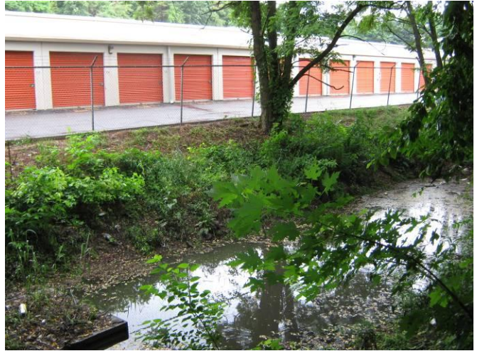
Overview of SWM facility from fence line
