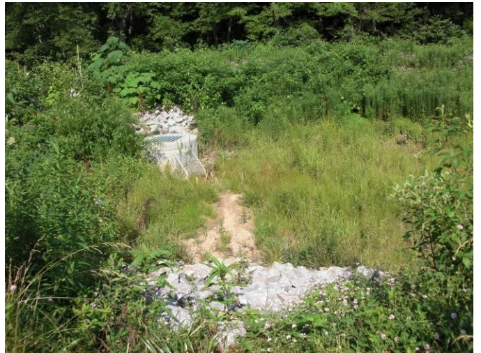
Overview of SWM facility from access gate
