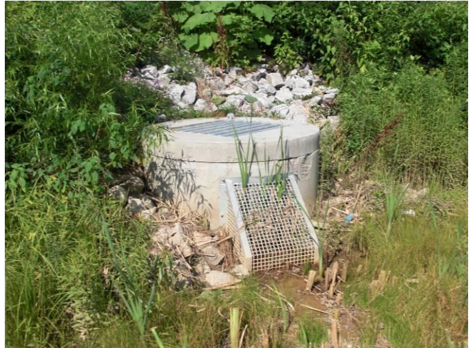
Overview of the outlet riser and low flow orifice
