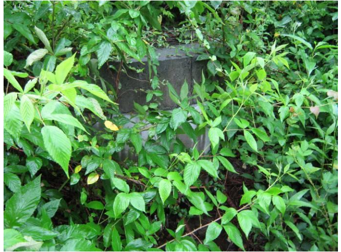
Overview of BMP outlet riser structure
