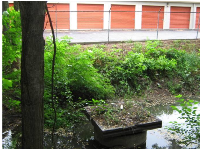
Overview of riser structure from fence line
