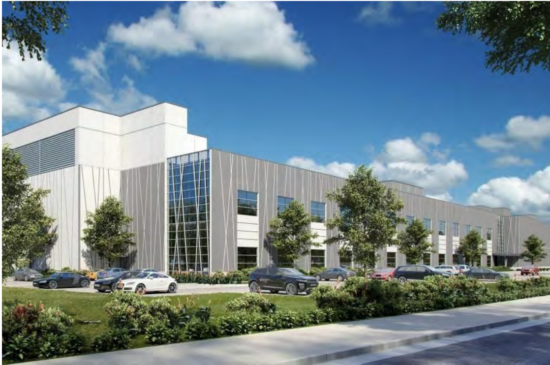
Modern architecture for Cloud HQ (Courtesy of Data Center Hawk)
