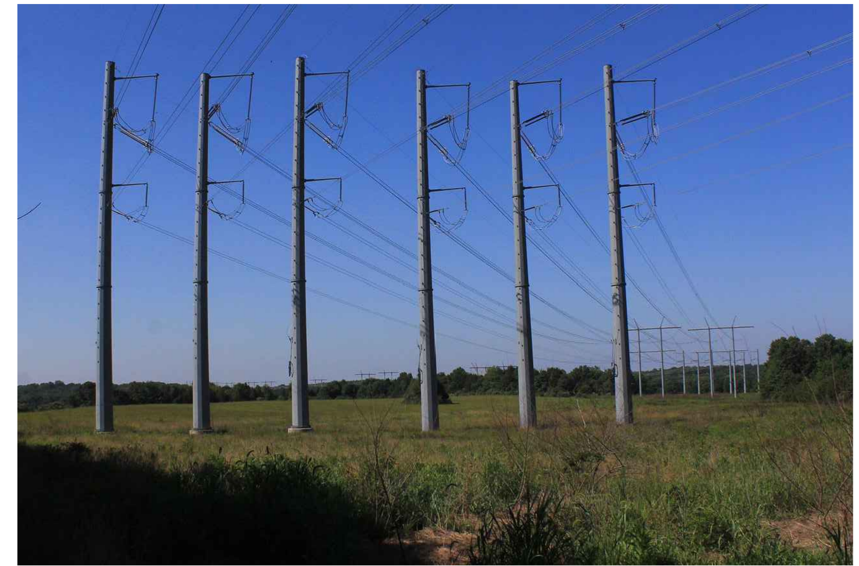
1 BRIDLE TRAIL (LOOKING SOUTHWEST)
