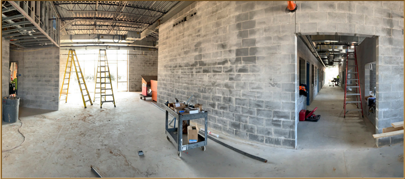
Construction progress at interior of Prince William County Animal Shelter
