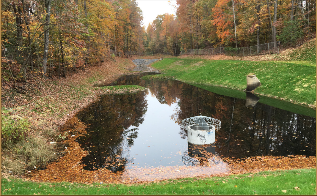
Powells Creek Watershed Water Quality Retrofit
