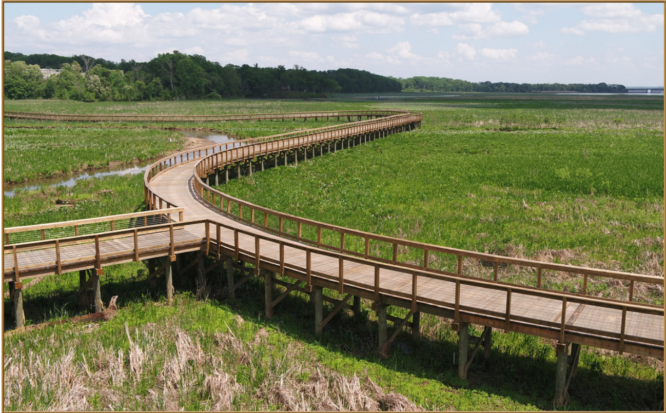
Neabsco Creek Boardwalk
