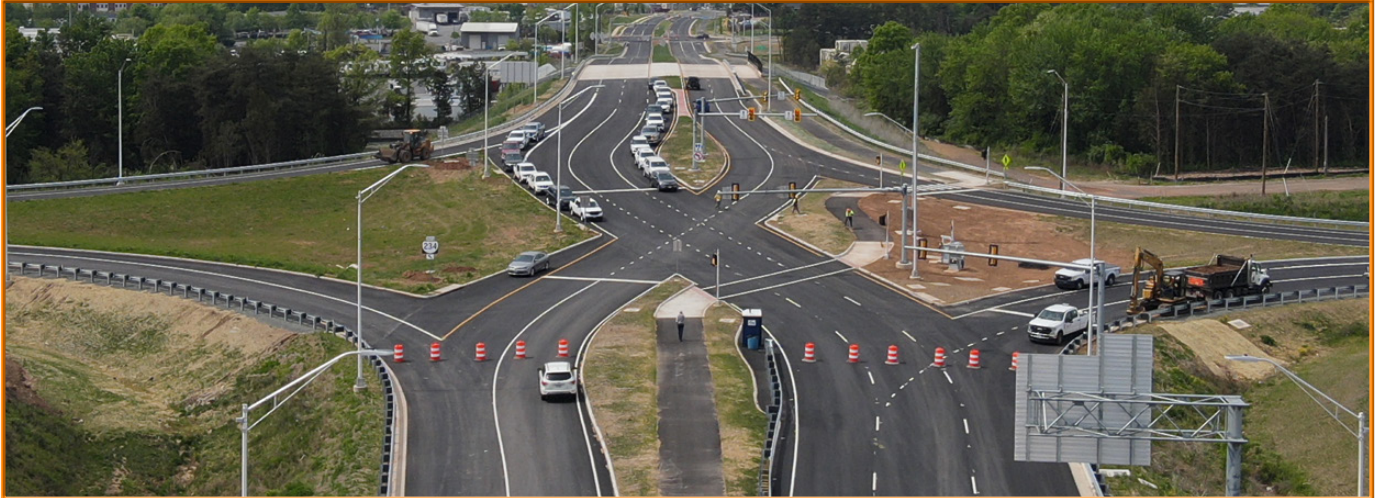
Balls Ford Road Interchange
