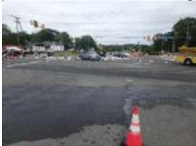
photos:Groundlevel overview looking westbound PWC Pkwy
