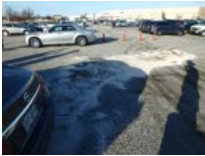
View of leak with absorbent, pads, and booms.
