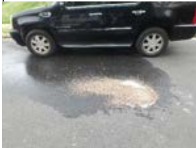
Spill in front of 4705 Kenny Court # 3
