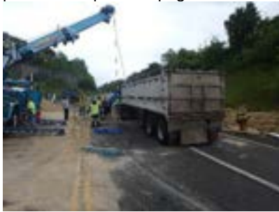
photos:Dump truck uprighted.
