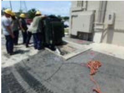
photos:NOVEC deployed absorbant socks
