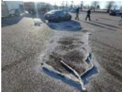
View #2 of leak with absorbent, pads, and booms.
