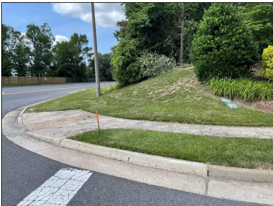
Photo 6: Buried Utilities and Grading along East Side of Devlin Road, Looking North.
