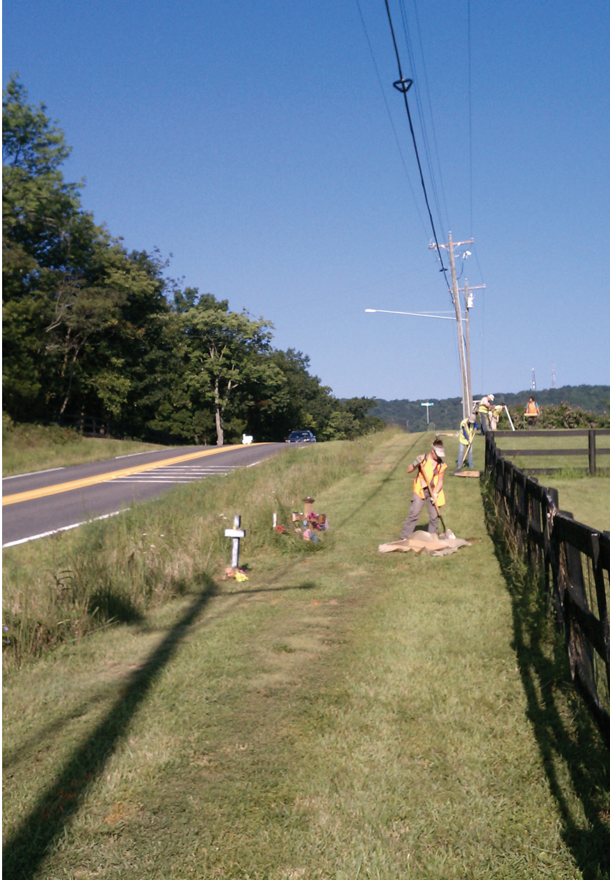
Figure 7. Logmill project corridor, view to west.
