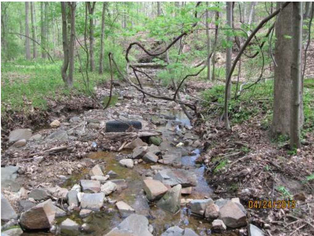
26. Looking downstream at a typical section of Stream Reach 8A. This stream is incised with erosion present along both banks.
