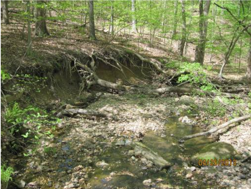
25. Looking downstream at a section of severely eroding bank at a stream bend in Stream Reach 7.
