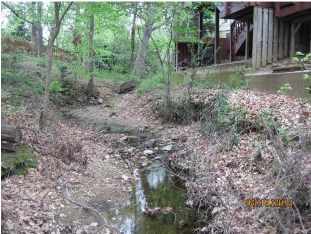
54. Looking upstream at a typical section of Stream Reach 17B. This section is eroding and unstable, and could pose a threat to the encroaching adjacent residences.
