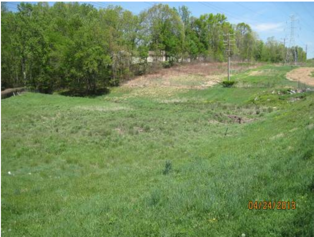
14. Looking across the stormwater management pond located on-line with Stream Reach 5.
