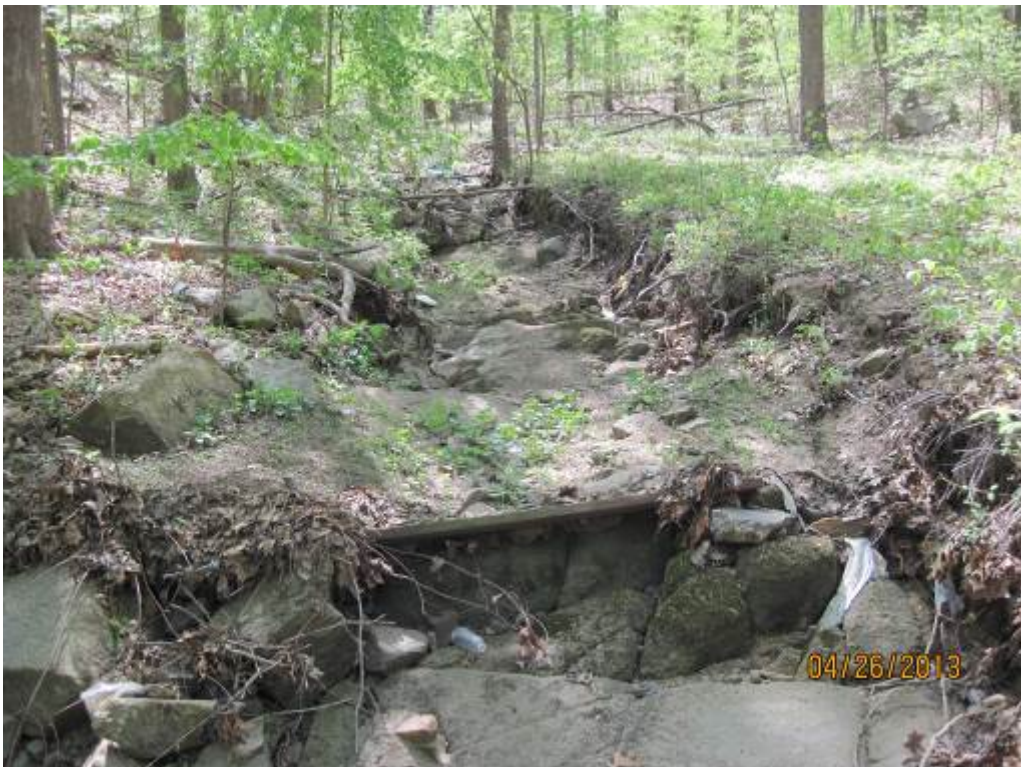
42. Looking upstream at a typical section of Stream Reach 12. Incision is present along most of this stream.
