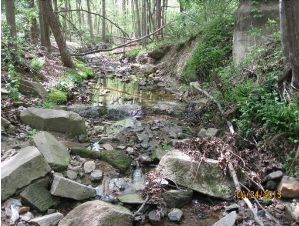
29. Looking upstream at a typical section of Stream Reach 8B. An exposed sanitary sewer line is present in this location, due to the increased incision and erosion occurring along this stream.
