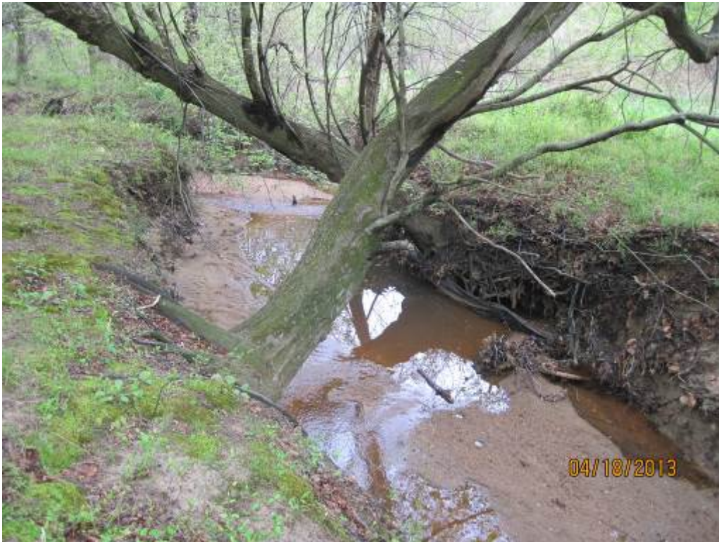
79. Looking upstream at a typical section of Stream Reach 23.
