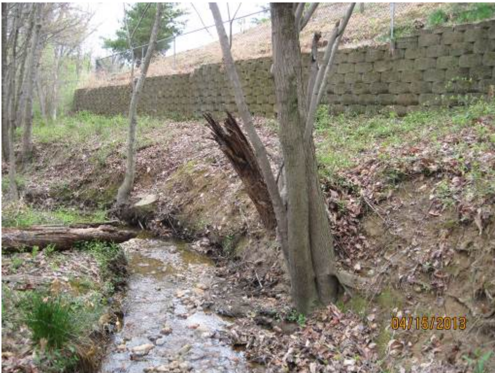
62. Looking downstream at a typical section of Stream Reach 19A. Residential encroachment along this stream has compromised the riparian zone.
