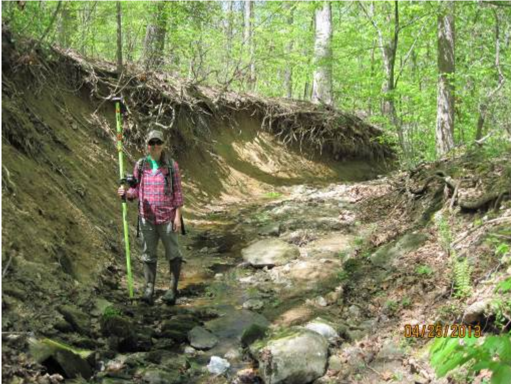
33. Looking downstream at massive erosion present along a section of Stream Reach 9.
