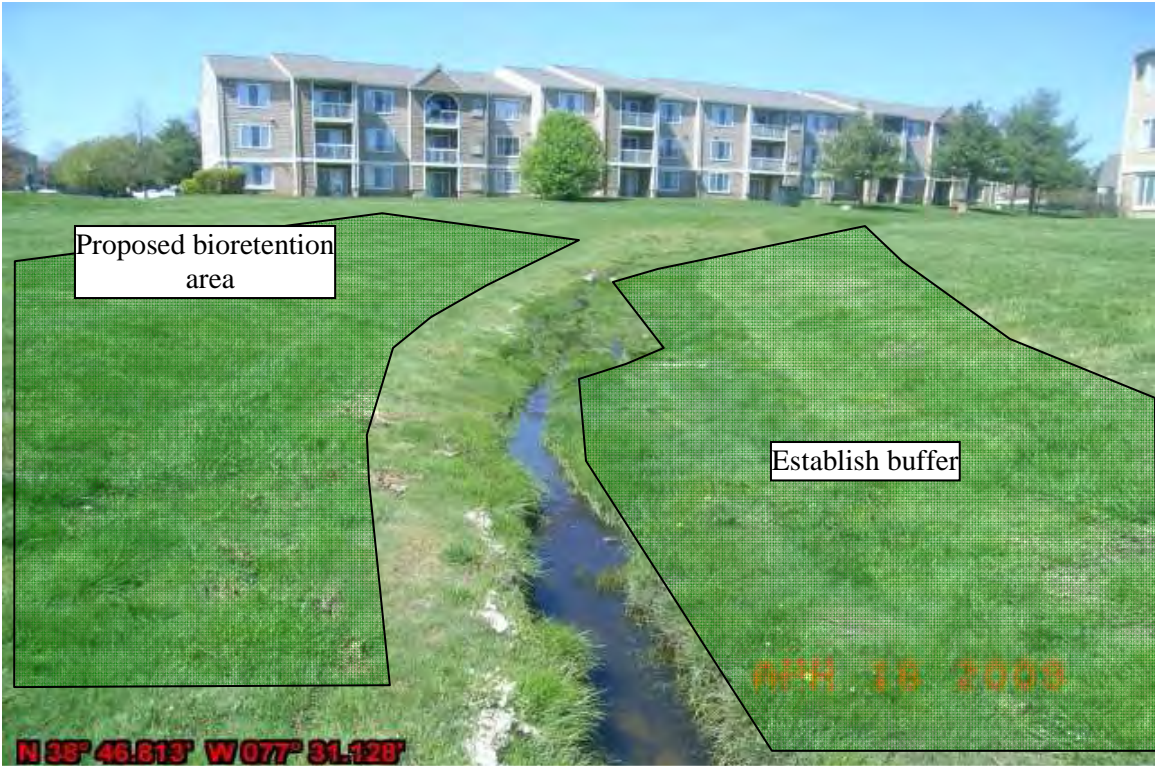
Photo 1: Drainage swale in common property would be converted to water quality BMP
