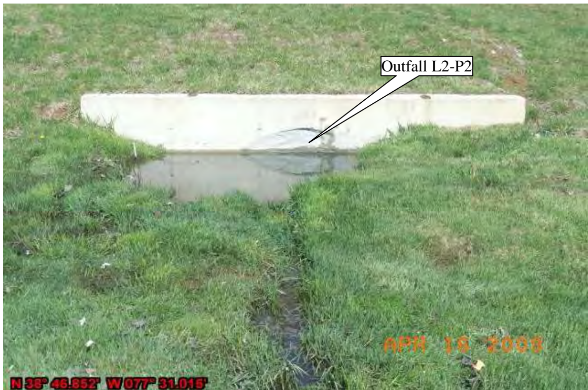
Photo 3: Outfall L2-P2 would be cleaned out
