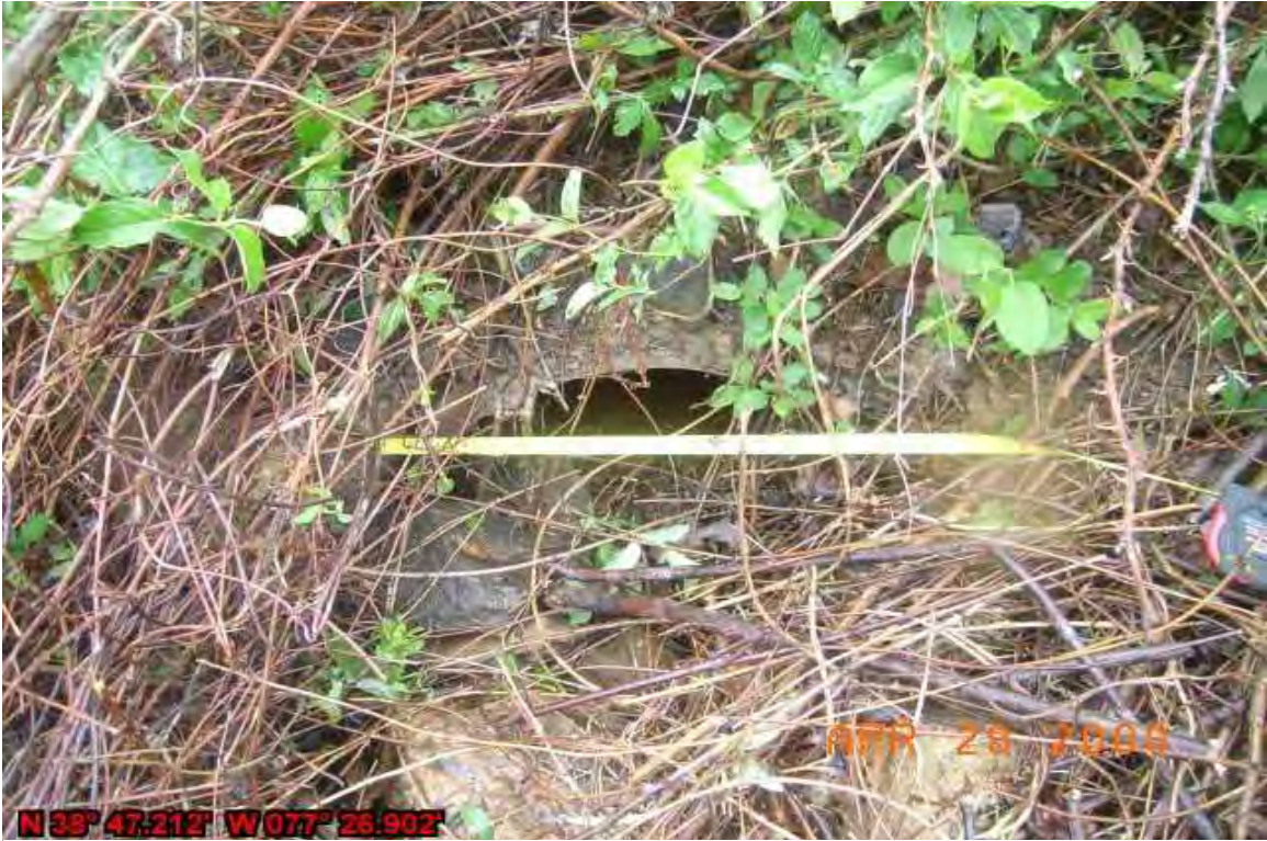
Photo 3: Remove sediments and debris from outfall Y7-P2
