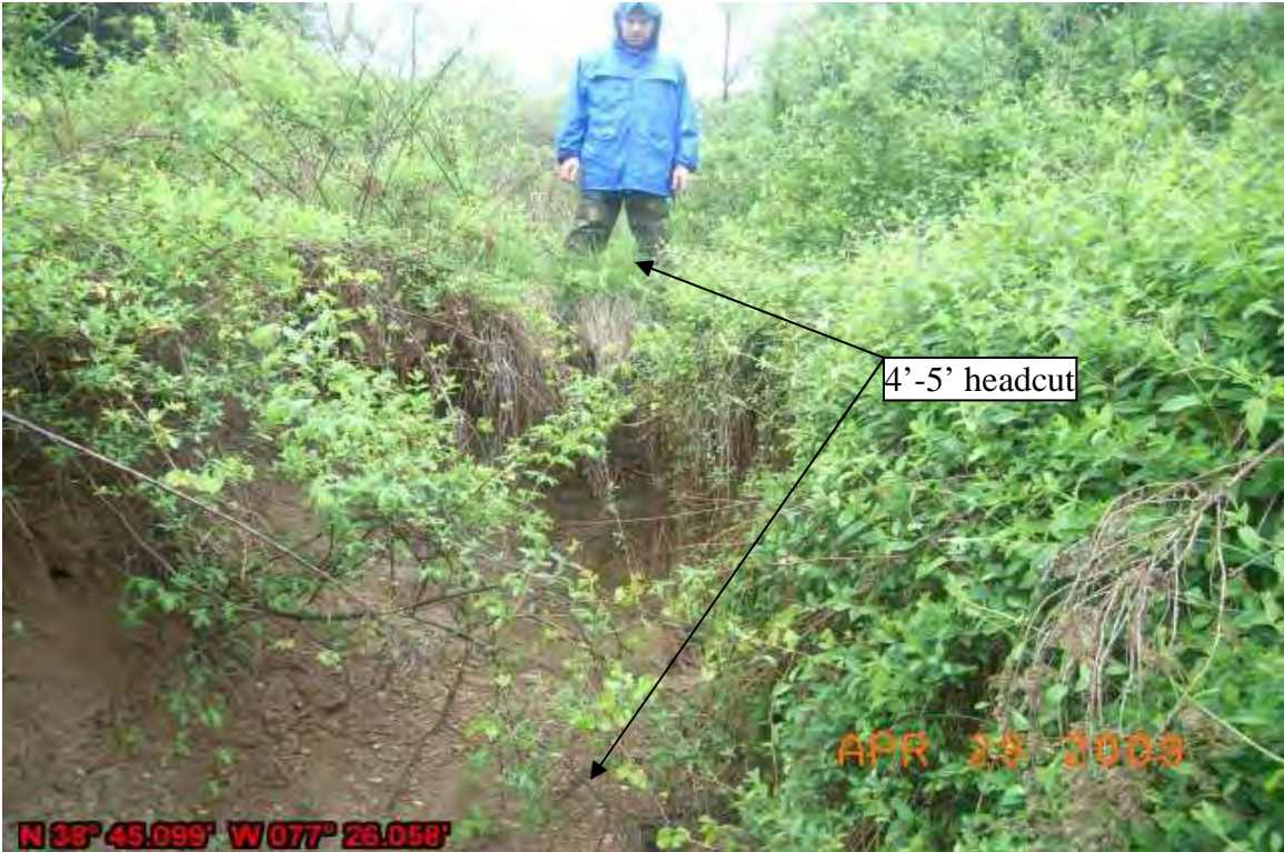
Photo 2: Headcut B6C-H2 would be stabilized
