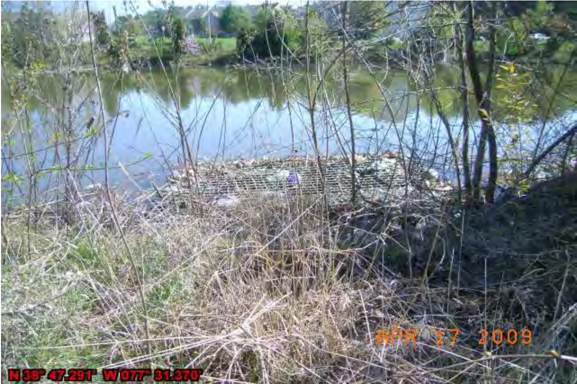
Photo 1: Existing 108 inch riser with flat debris grate
