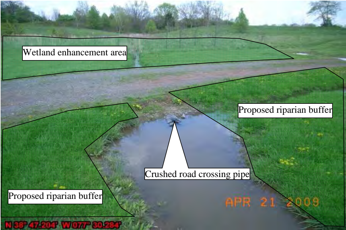
Photo 1: Replacement of crushed pipe
