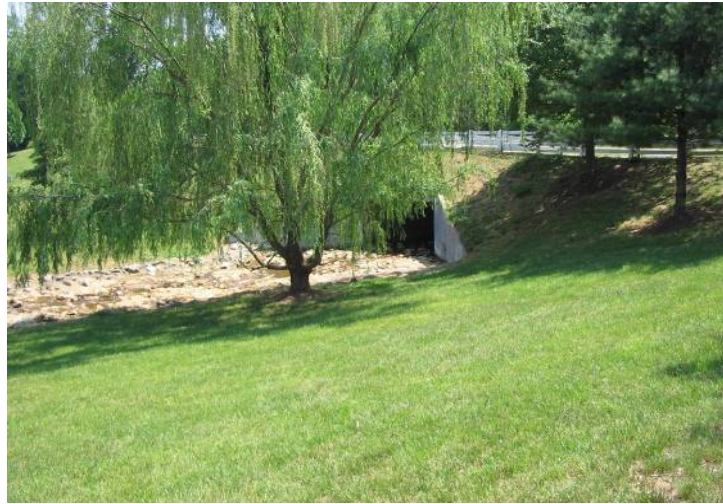
Downstream face of culvert under Powells Creek Boulevard
