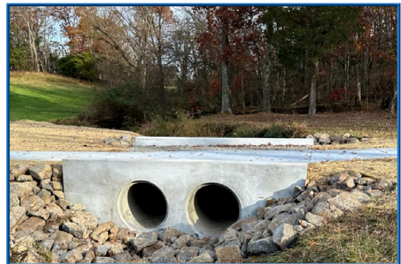
Prince William Golf Course Culvert Repair
