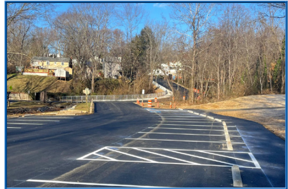
Cloverdale Park Site Improvements
