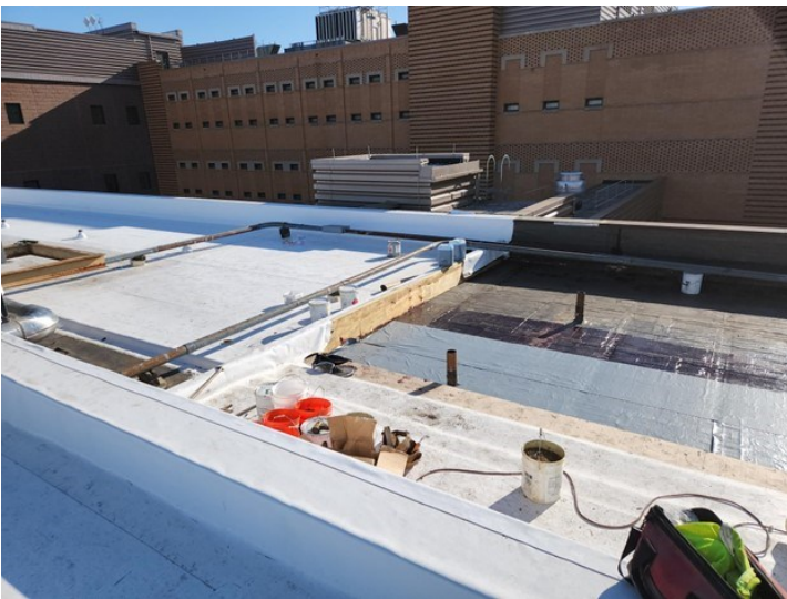
Main building roof during repairs
