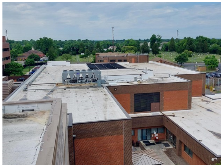
Main building roof completed
