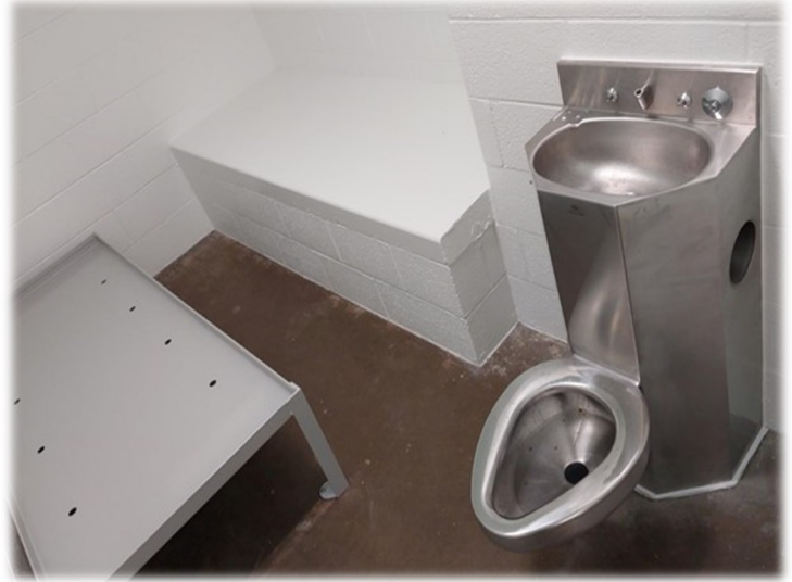
Refurbished inmate cell
