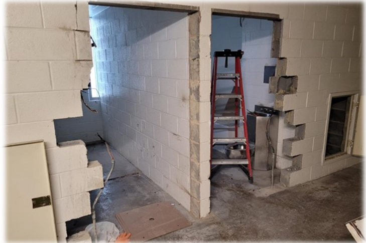
Repairs to inmate cell doors
