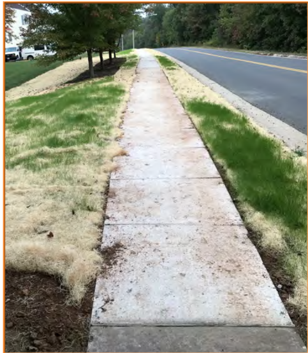
Godwin Drive Sidewalk – This project completed a missing section of sidewalk on Godwin Drive adjacent to Lancaster Knoll Lane.
