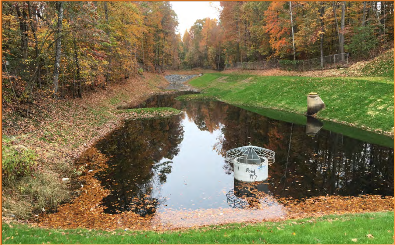
Powells Creek Watershed Water Quality Retrofit
