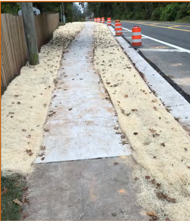
Lucasville Road Sidewalk – This project completed a missing section of sidewalk on Lucasville Road adjacent to Lomax Forest Drive.
