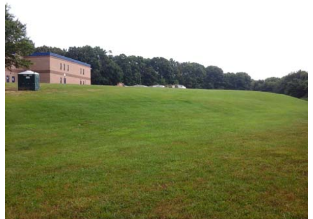
View looking northeast through site UFOR119.
