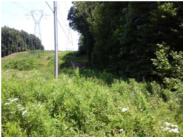
View looking northeast through the electric transmission line ROW at site UFOR137
