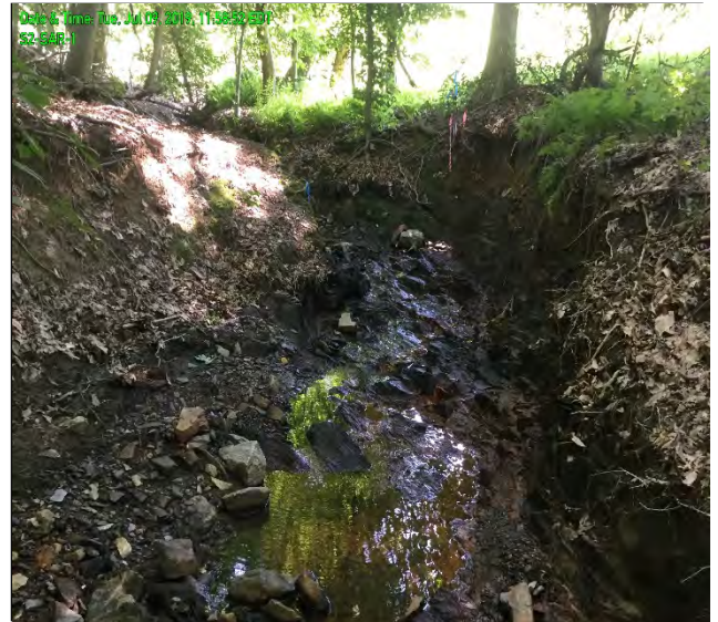
Photo 18: Upper reach of Stream 2/Stream B. Scored intermittent. Highly scoured/incised.
