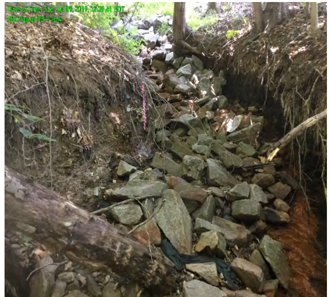
Photo 20: Stream 2/Stream B at buried channel by riprap. Scored intermittent.
