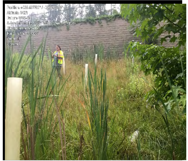
Photo 14: Upslope view of man-induced feature and FDP 5. Retaining wall in background.
