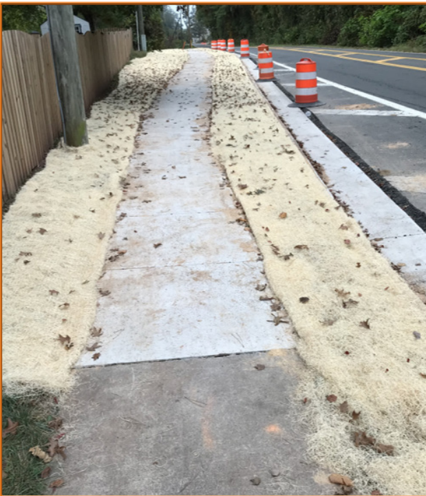
Lucasville Road Sidewalk – This project completed a missing section of sidewalk on Lucasville Road adjacent to Lomax Forest Drive.
