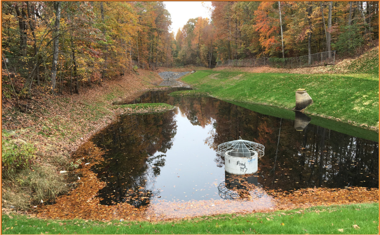
Powells Creek Watershed Water Quality Retrofit
