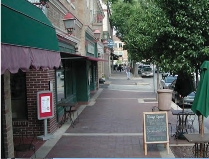
Driveway across sidewalk identified by material change.
