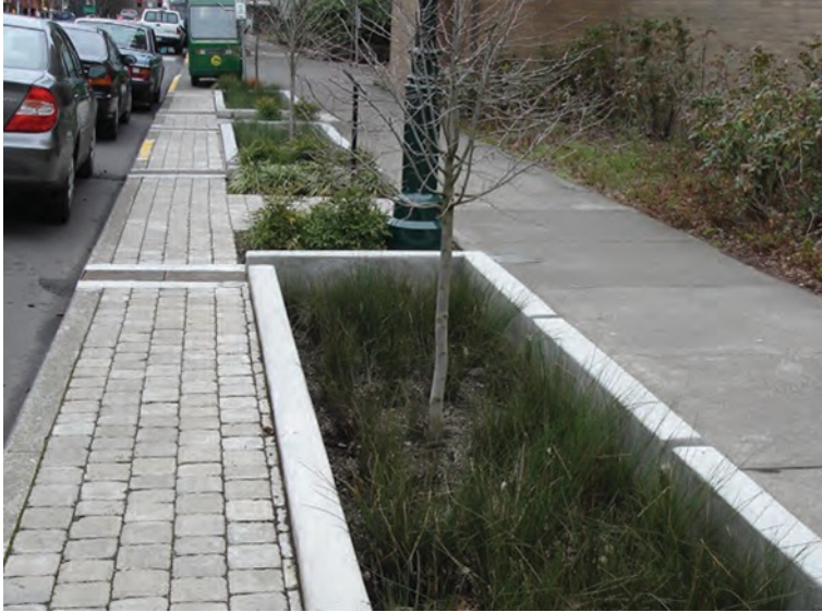
Low impact development (LID) curbside planting strips creating a buffer between the roadway and the sidewalk.
