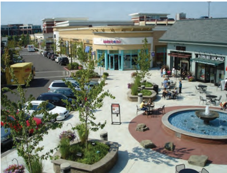
Façades and entries oriented towards plaza.
