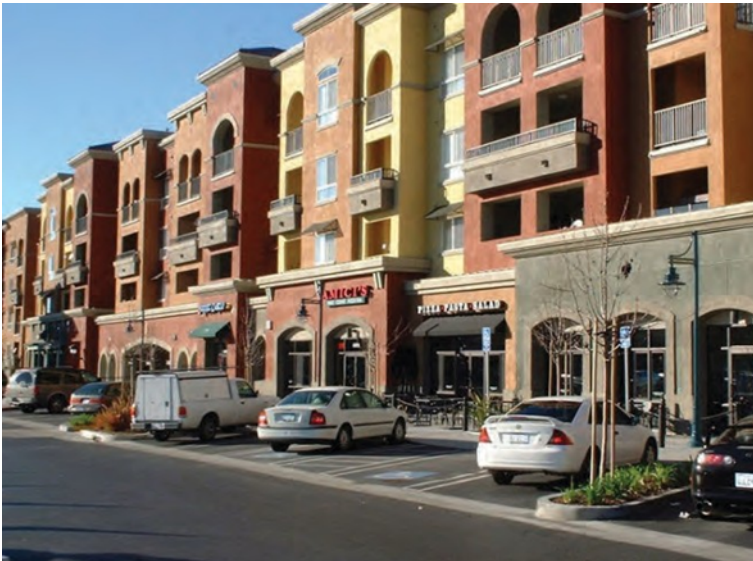
On-street diagonal parking.
