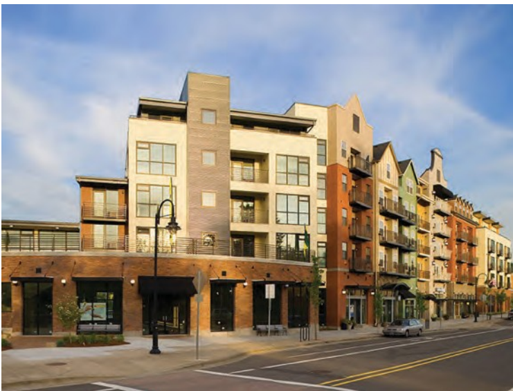
Vertical articulation of buildings.
