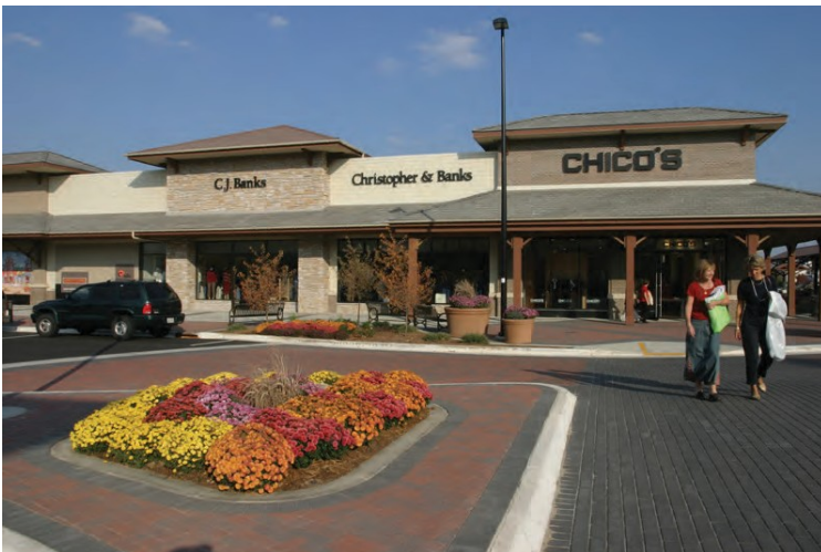
Example façade of a one-story building that includes vertical and horizontal modulation.
