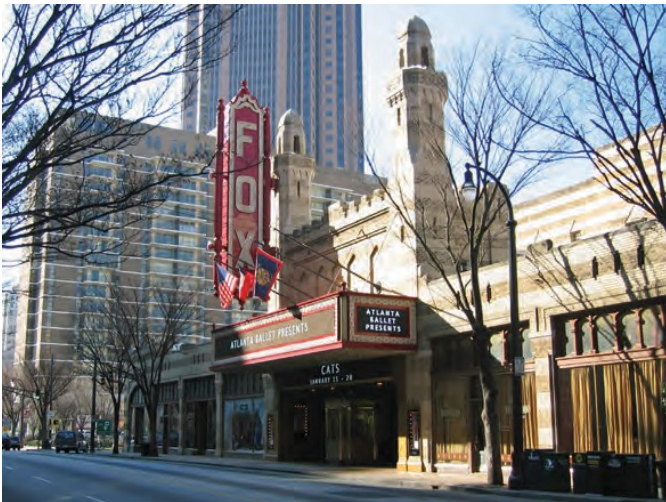
Primary building entry oriented towards street.
