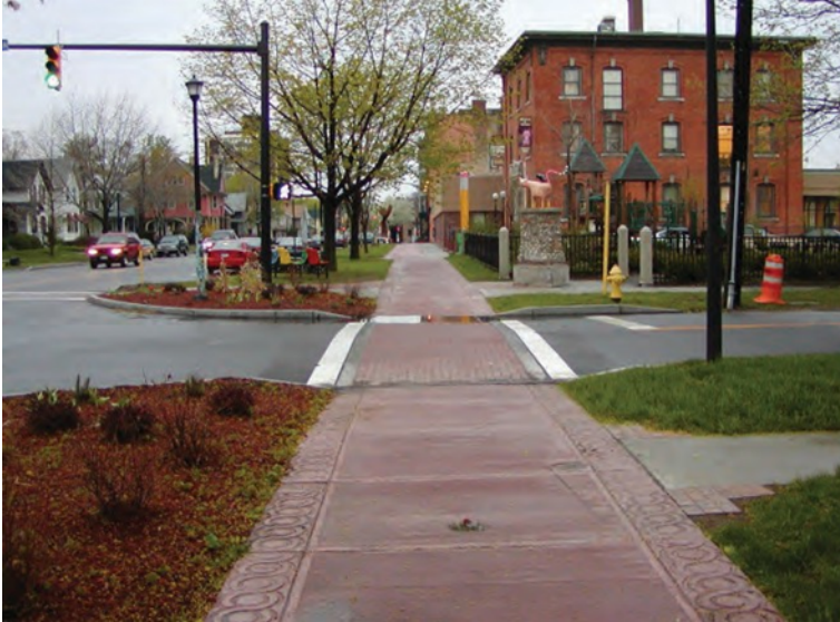
Special paving material and pattern used for sidewalk and crosswalk paving.
