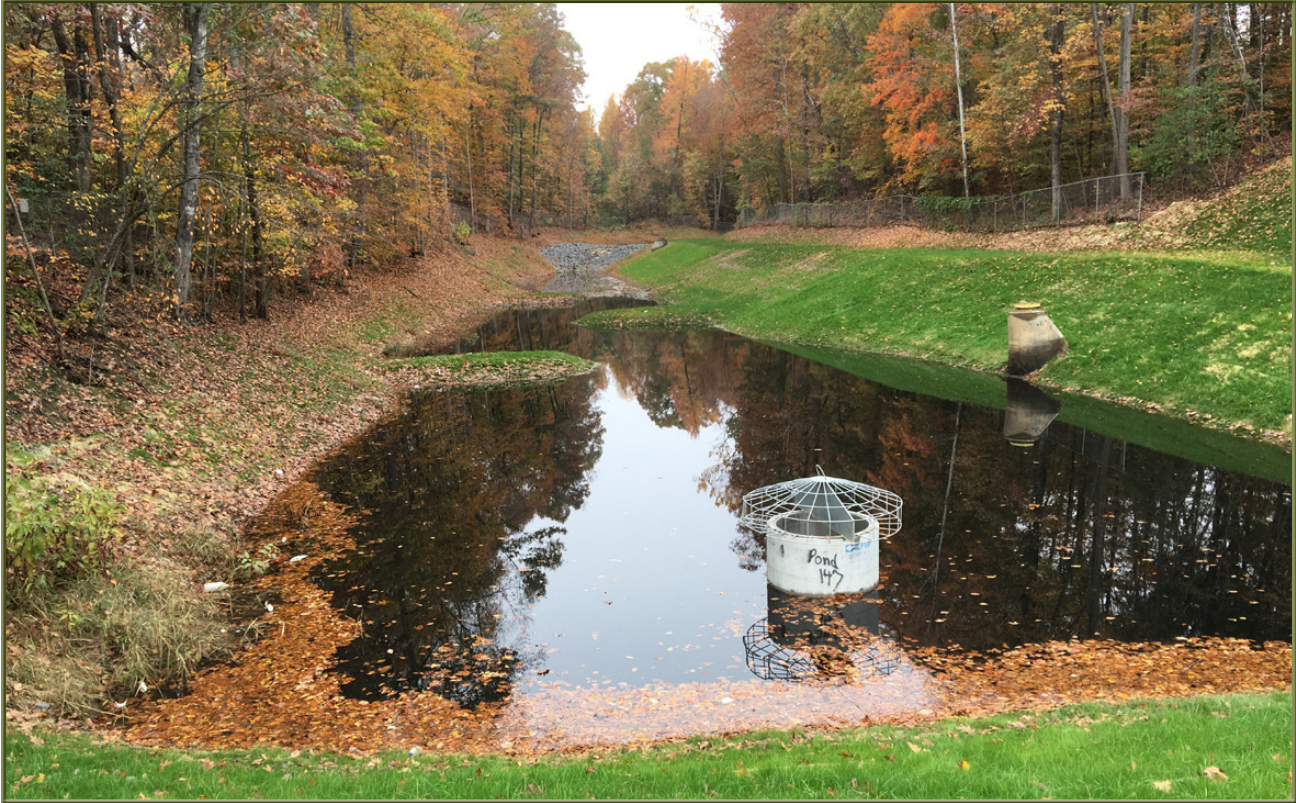
Powells Creek Watershed Water Quality Retrofit
