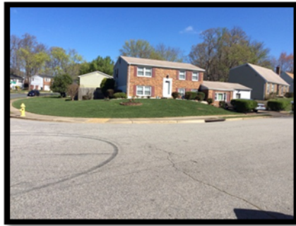
Inlet-1 in front of property 13816
