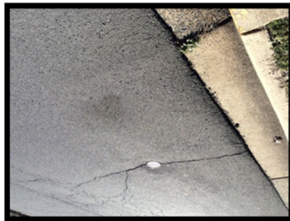
Water Main control valve
