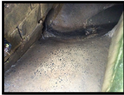
Inlet-4(across the Street)
