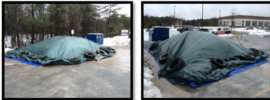
Properly covered & no contact with flowing water
