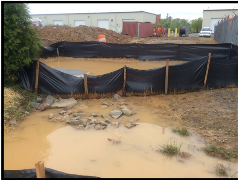
Zone -2 (Silt fence around outlet –Double step with additional Straw Bale Barrier)
