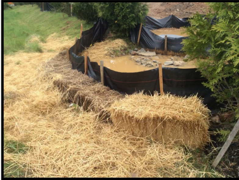
Zone -2 (Silt fence around outlet –Double step with additional Straw Bale Barrier)
