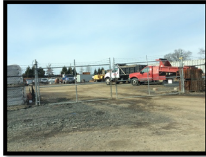
Parking Vehicle & Construction Materials
